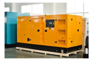
Dimension:3600\*1600\*1900mm Weight:3600kg Fuel Tank:550L
