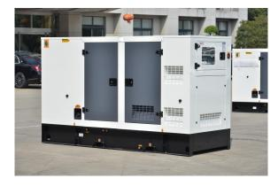
Dimension:3000\*1100\*1700mm Weight:1700kg Fuel Tank:280L
