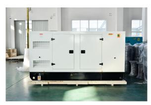
Dimension:3600\*1600\*1900mm Weight:3150kg Fuel Tank:550L
