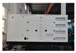
Dimension:5200\*2100\*2500mm Weight:9700kg Fuel Tank Capacity:1000L
