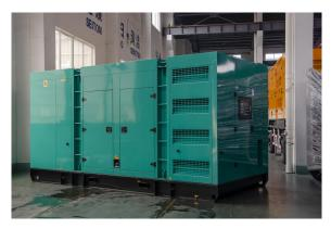
Dimension:4700\*2100\*2400mm Weight:6800kg Fuel Tank Capacity:1000L
